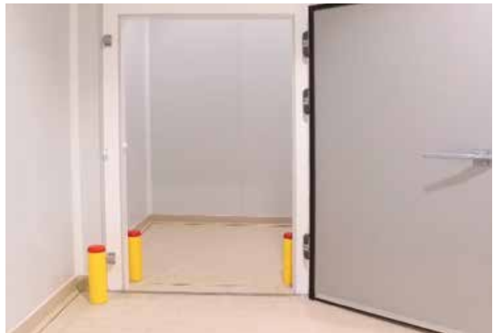
Bollards for protection of shelves and doors
